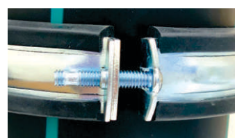
Upper sliding clamp tightening level
